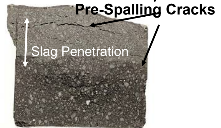
Brick from Side Wall
